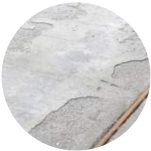
Spalled Concrete
